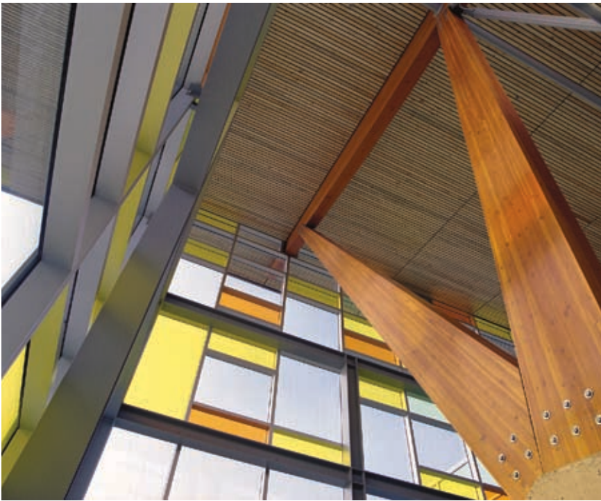
Above: The atrium consists of eye-catching, multi-coloured glazing and interior glulam beams. Wood products used in the structure contain no added urea formaldehyde resins.
