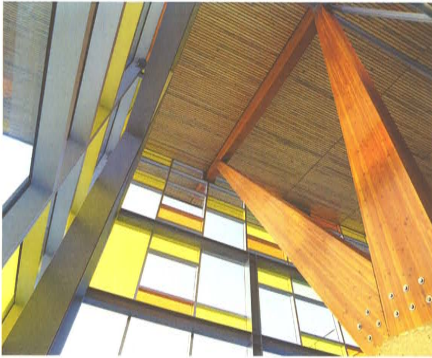
Above: The atrium consists of eye-catching, multi-coloured glazing and interior glulam beams. Wood products used in the structure contain no added urea formaldehyde resins.
